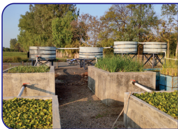
Weed-based phytoremediation system developed at ICAR-DWR and irrigation of vegetables through treated water
